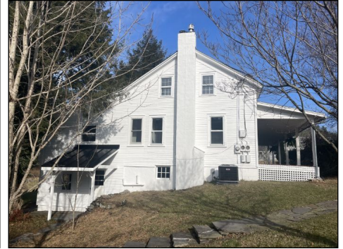
Left side of the building
