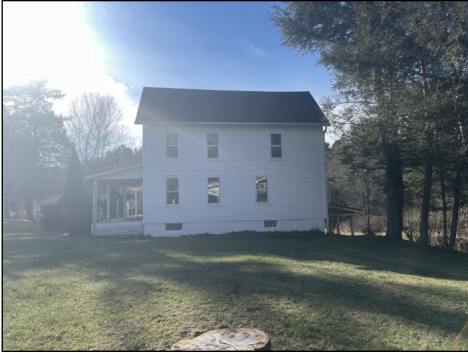
Right side of the building
